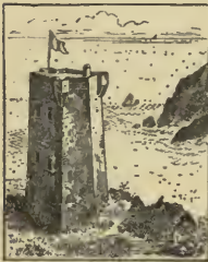
DEFENCE TOWERS, CO. DONEGAL.
